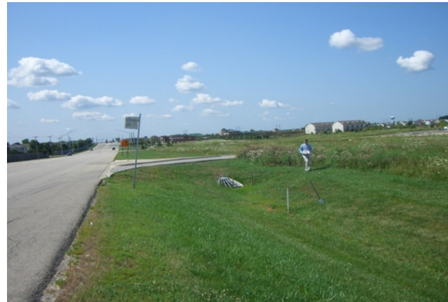
Route 529 bus stop without landing and walkway
