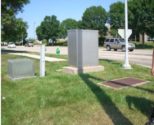
Signal equipment blocking extension of sidewalk, SW corner Randall & McKee St., view NW
